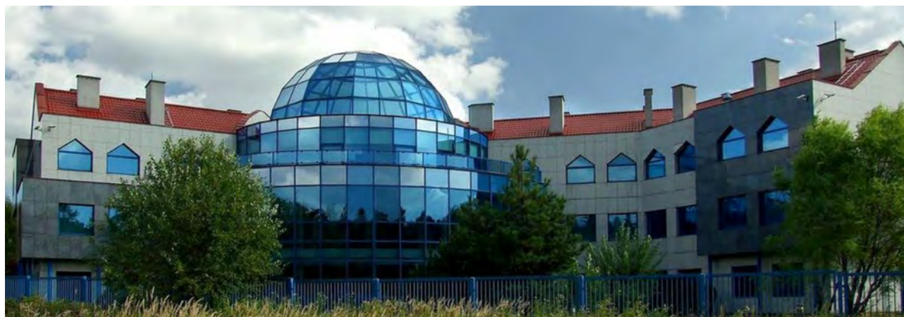
Fig. 2. General view of the CUS building in Psary
