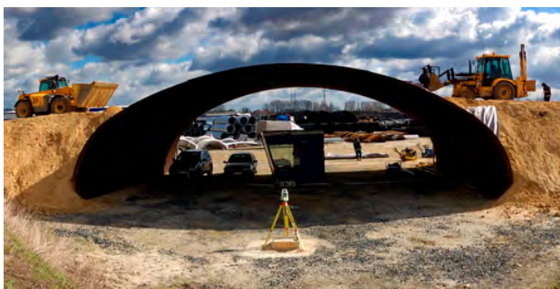
Fig. 4. The SuperCor SC-57S structure during construction
