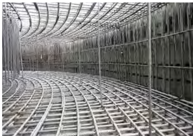
Fig. 7. Reinforcement made of stainless steel [14]
