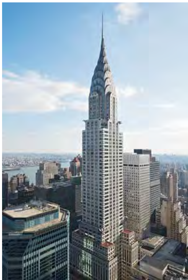
Fig. 1. Chrysler Building [7] Rys. 1. Chrysler Building [7]
